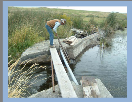
The Araujo Dam presented a major problem for spawning Coho Salmon. The flashboard dam has been removed and replaced by pump diversions. Photo Credit: US Fish & Wildlife Service Photo
