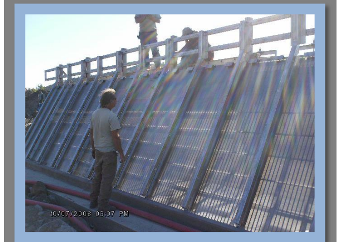
Installation of the fish screen panels. Photo Credit: SVRCD
