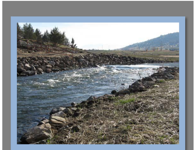
Post-Project: Dam removal with installed boulder weir. Photo Credit: SVRCD
